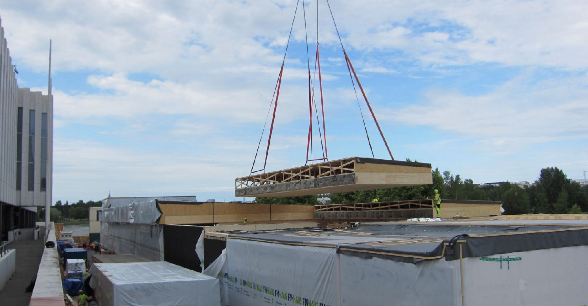
Roof elements were installed on site. Helsinki, 06/2021. Pikku-Finlandia
