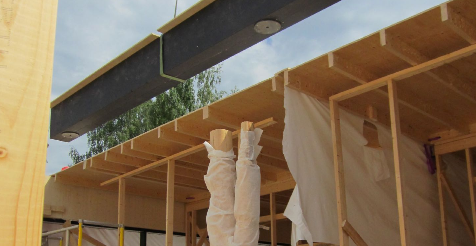
GL beams were installed on site. Helsinki, 06/2021. Pikku-Finlandia
