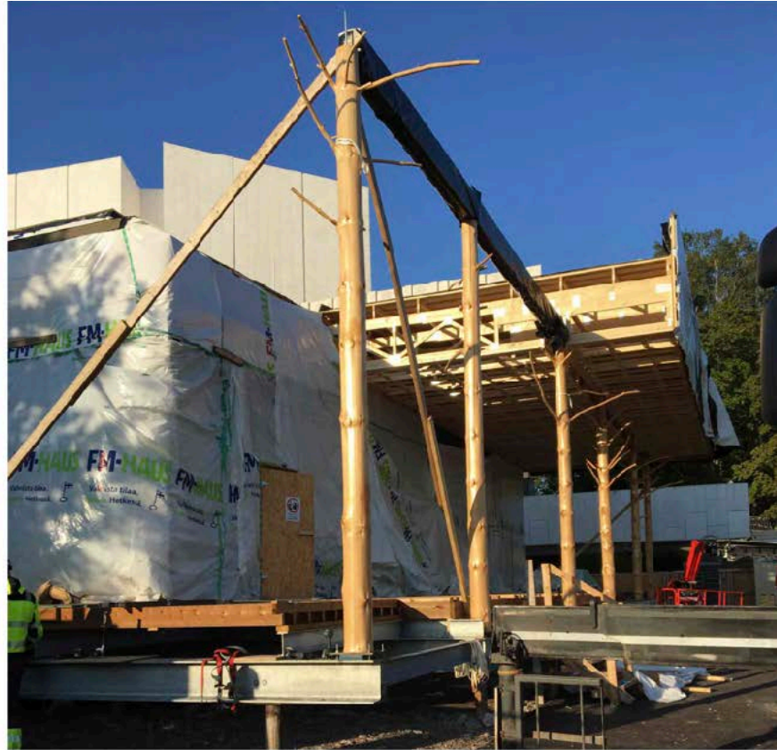
Columns which were not pre-installed in the volume elements were installed on site. Helsinki, 08/2021. Pikku-Finlandia
