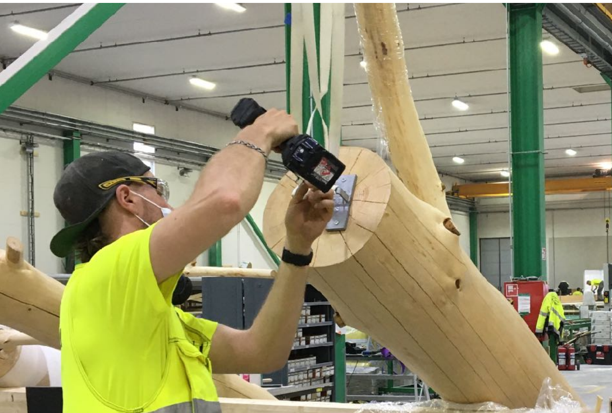
Tree-columns were pre-installed in volumetric modules by FM Haus. Jokioinen, 04/2021. Pikku-Finlandia
