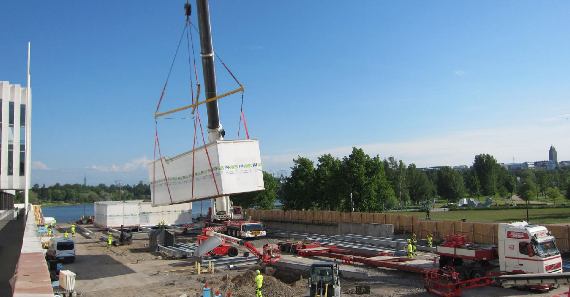
Prefabricated modules were transported to site. Helsinki, 05/2021. Pikku-Finlandia
